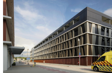
Parking Garage - Reinier de Graaf Hospital Delft
